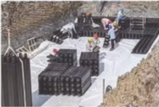
Step 4: Place the PP module
