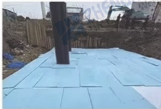
Step 8: Place the extruded board
