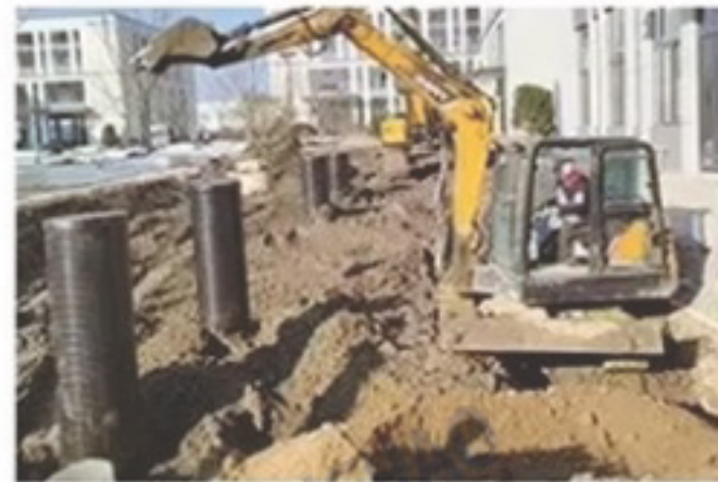
Step 9: Backfilling
